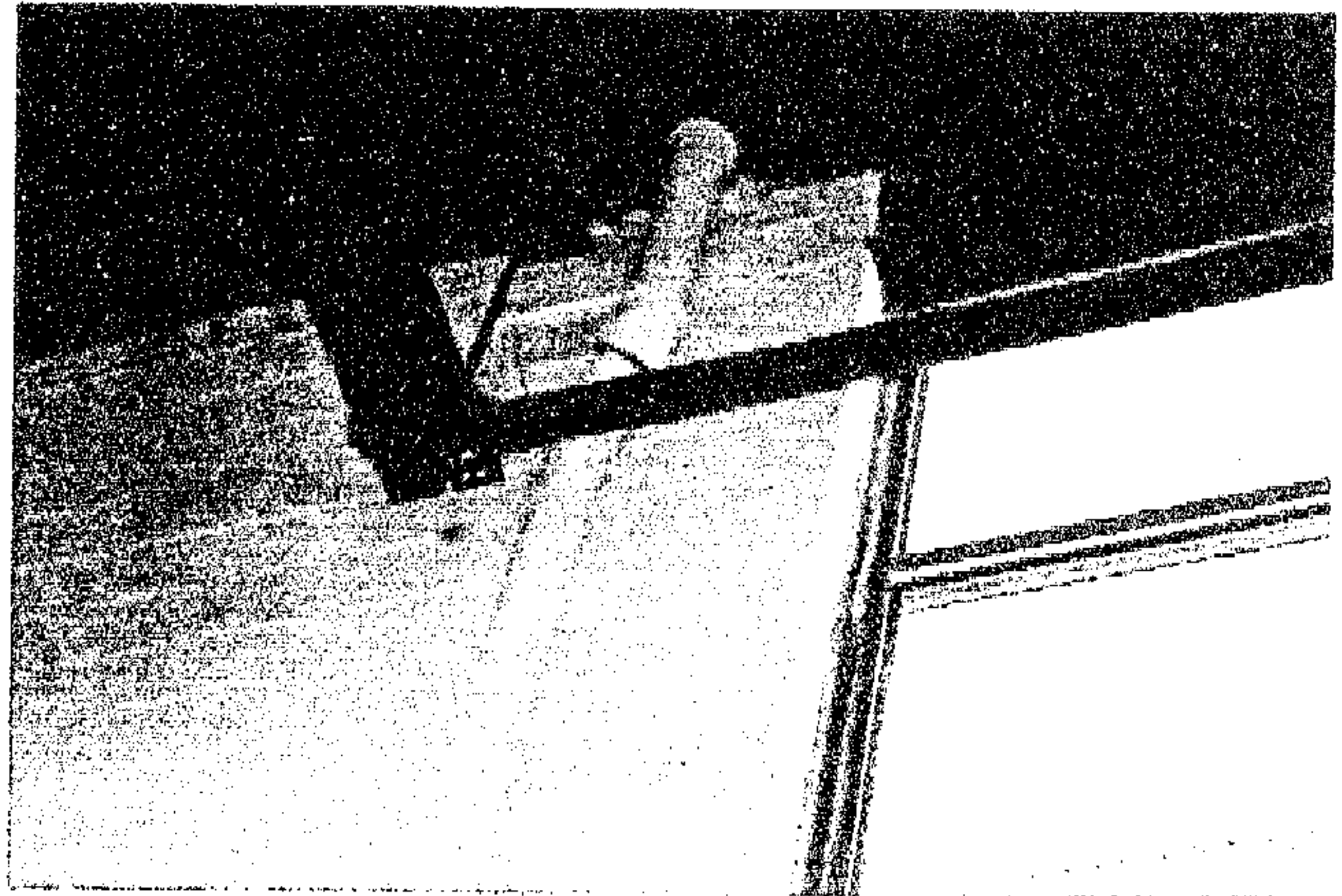
4. Gymnasium joist with bearing shear fracture.
